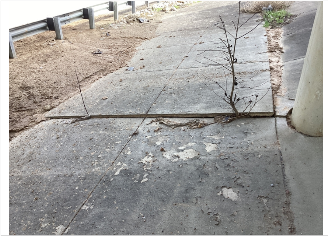
Tree growth between slope paving
