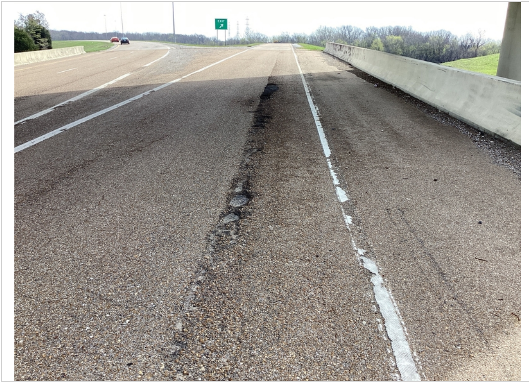
Top deck span #2 spalling
